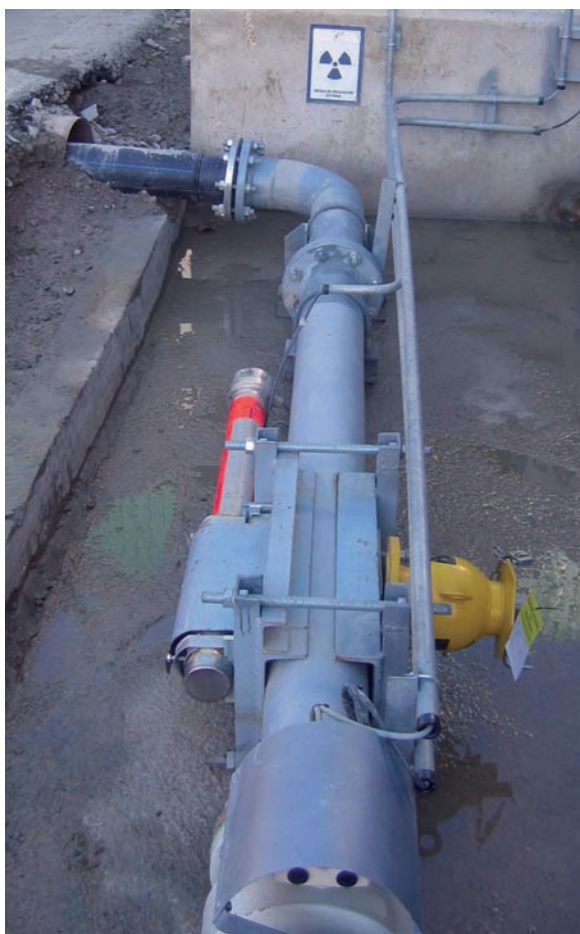
Control of processes for the measurement of the density of fluids flowing through piping.
