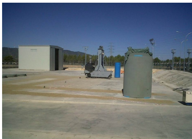
Ascó Nuclear Power Plant ITS facility.
