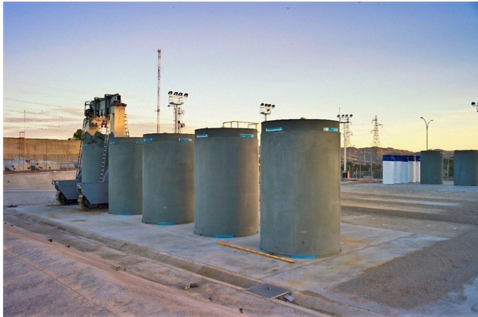
Image of the Individualised Temporary Storage at the Ascó nuclear power plant.
