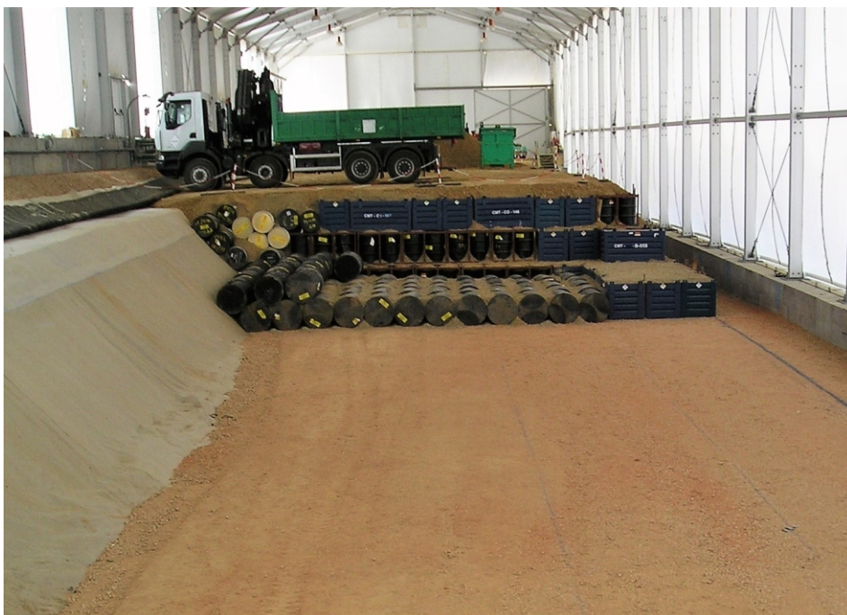
Image of the interior of the VLLW disposal cell at El Cabril.
