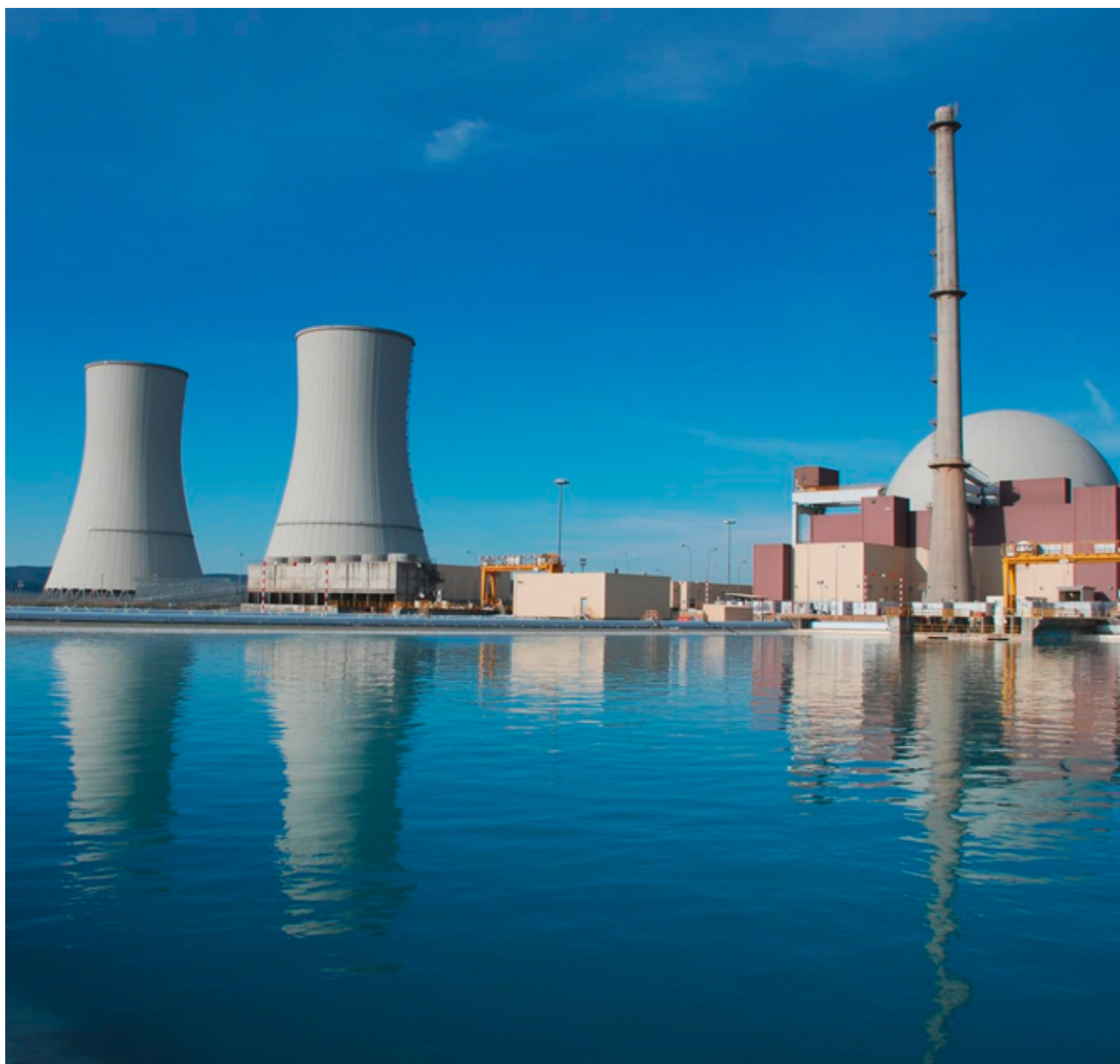
Figure 2. Trillo nuclear power plant
