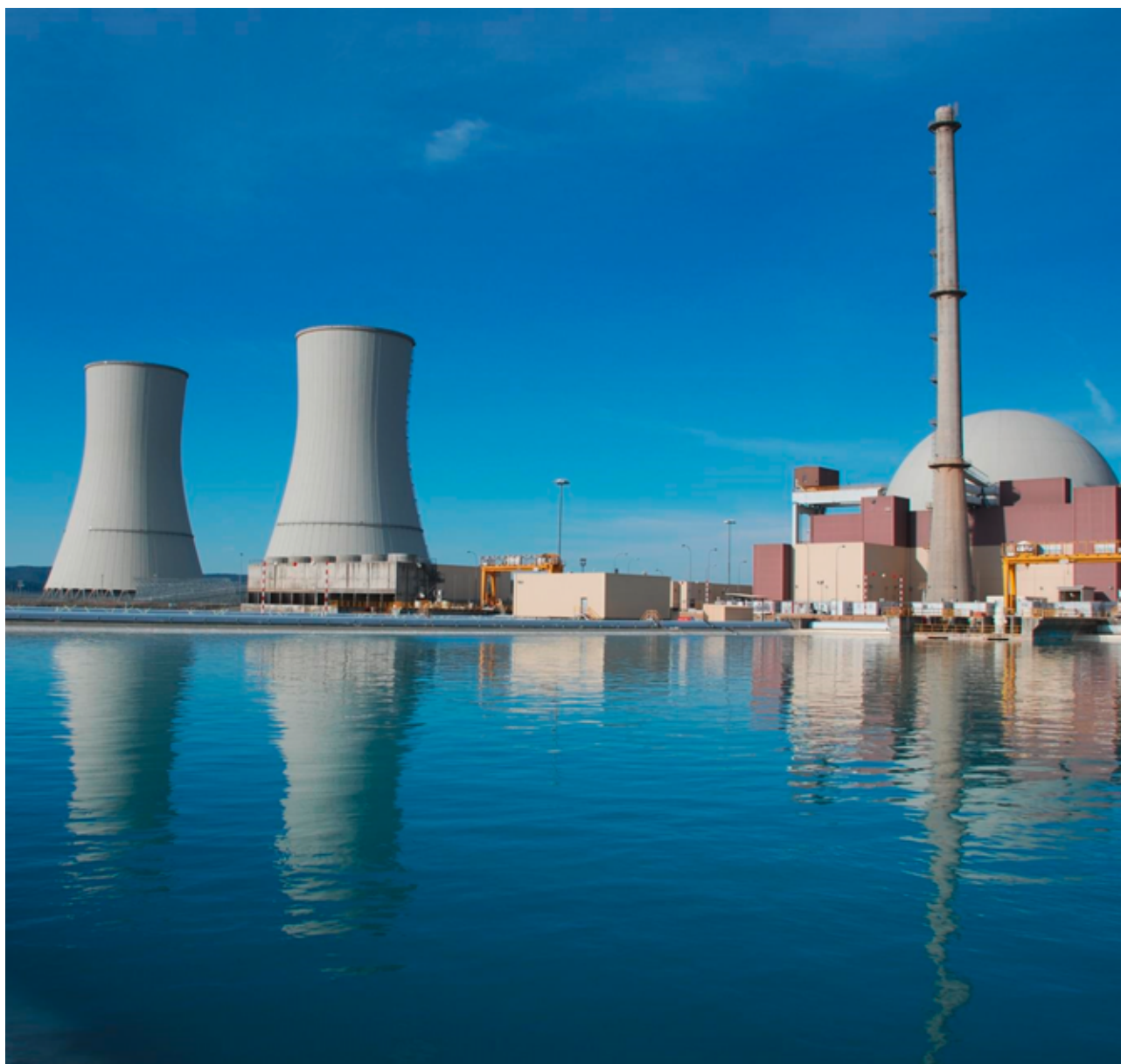
Figure 2. Trillo nuclear power plant
