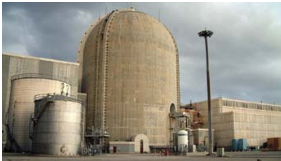
Central nuclear Vandellós II.
