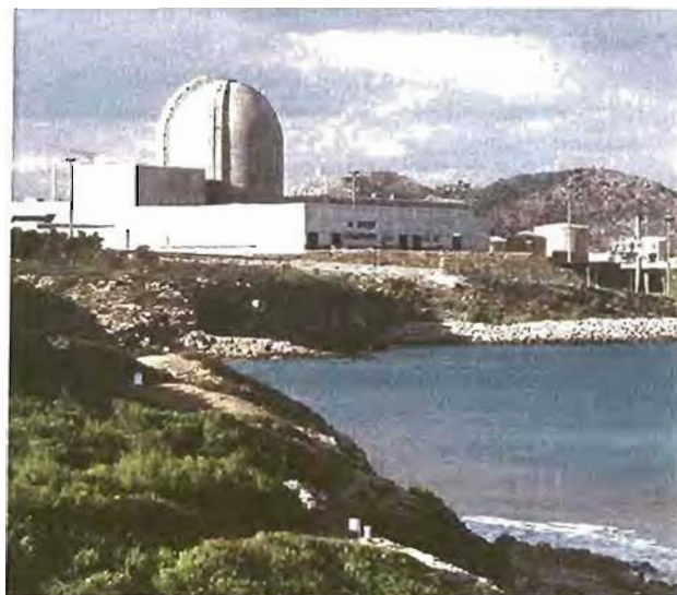
Central nuclear Vandellós II.
