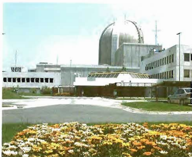
Central nuclear Vandellós II.
