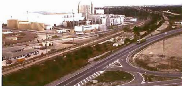
Central nuclear Vandellós II.
