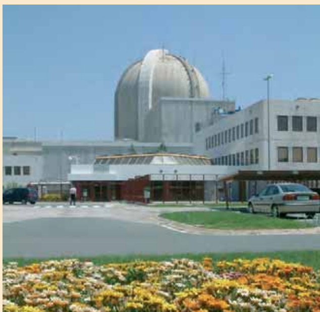
Central nuclear Vandellós II.
