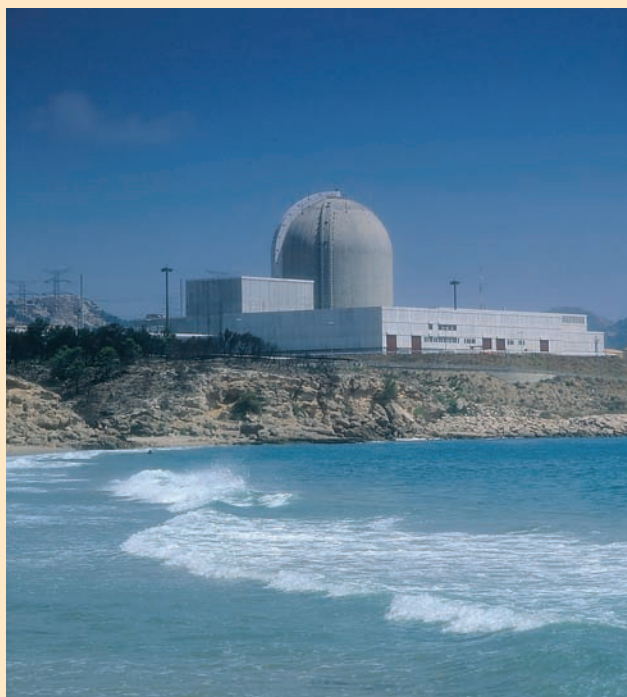
Central nuclear Vandellós II.
