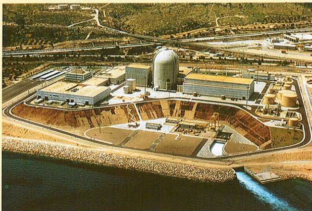
Central nuclear Vandellós II.
