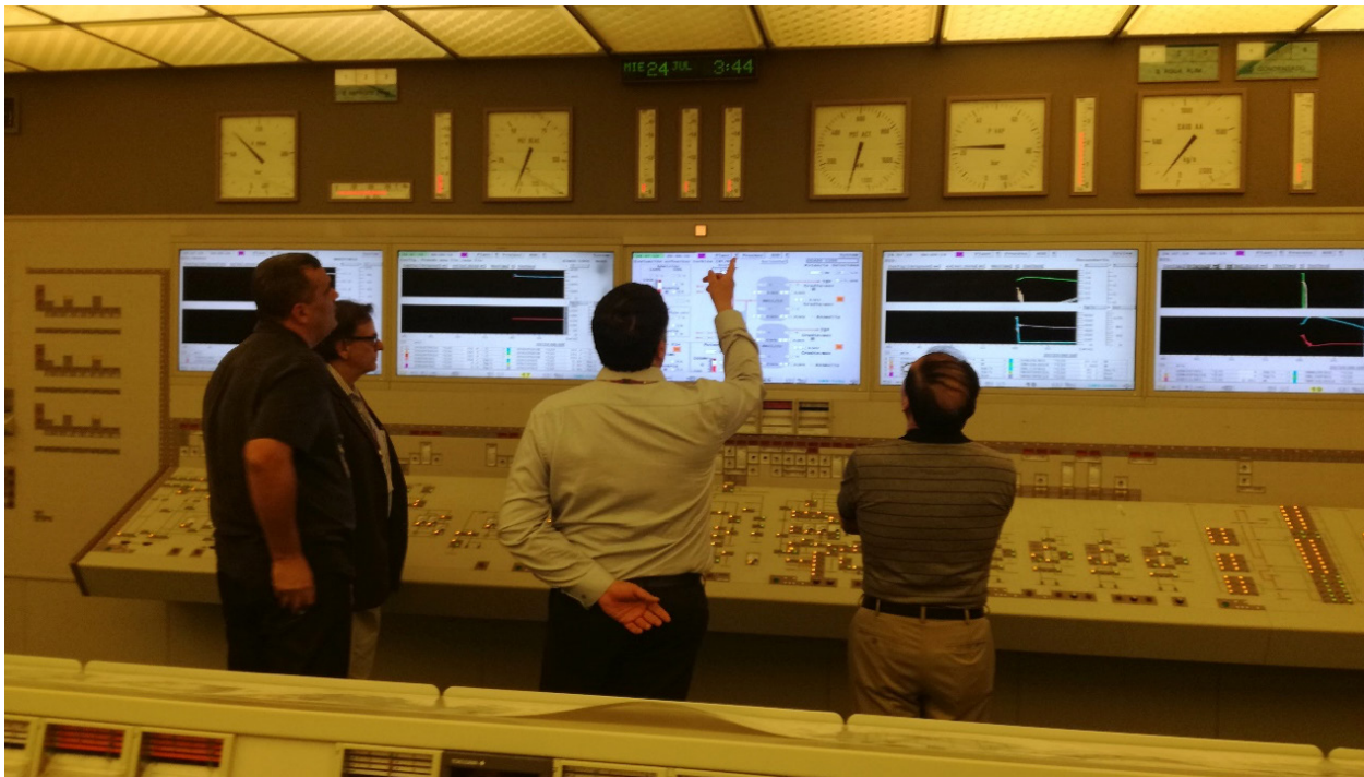
Technical visit of CLOR project experts to the control room at the Laguna Verde Nuclear Power Plant, Mexico
