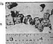
void inside of rubble bed.
