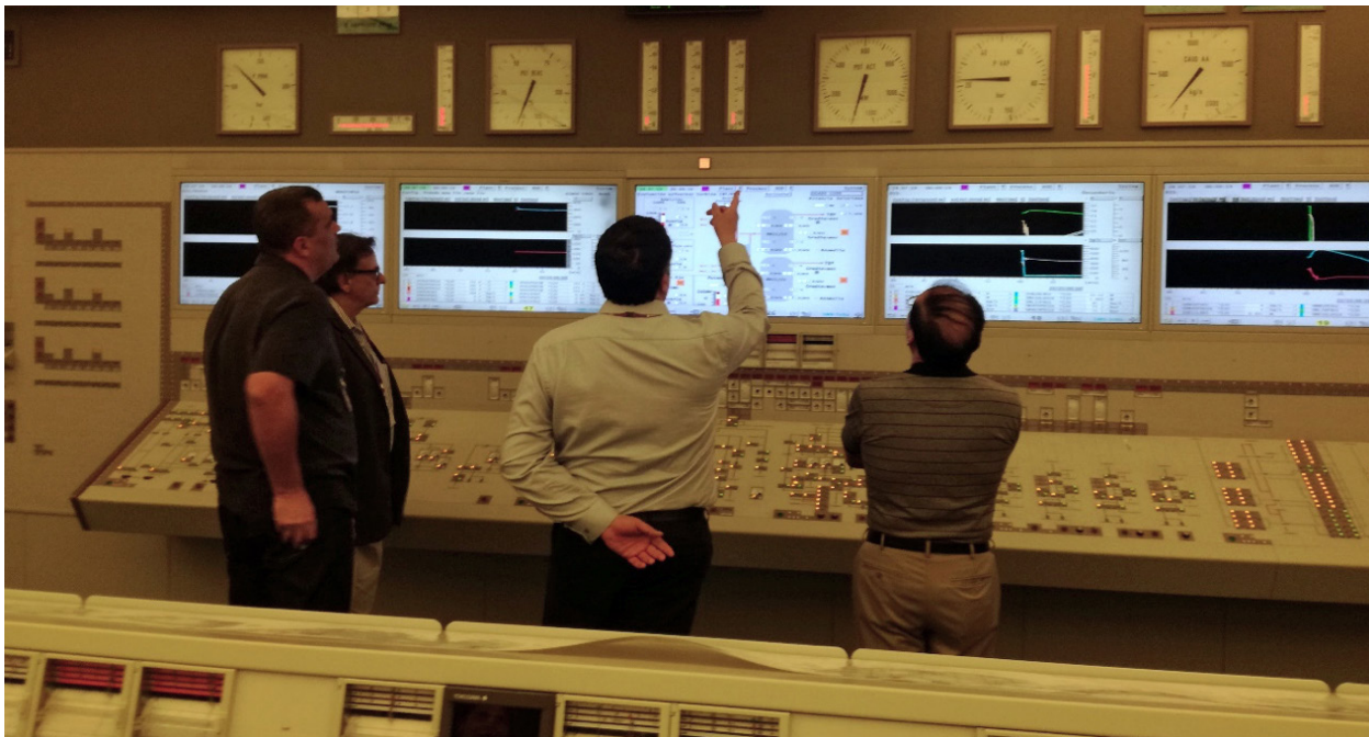
Technical visit by CLOR project experts to the control room of the Laguna Verde Nuclear Power Station, Mexico.
